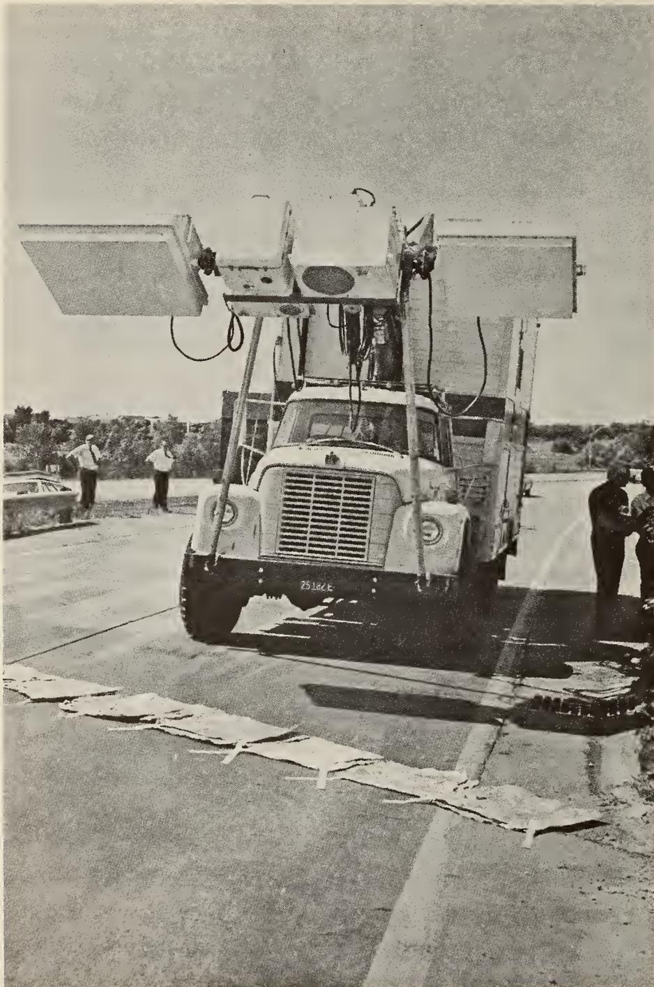
Figure 2.1 AGC's Microwave Mobile Field Laboratory at the Topeka, Kansas Bridge Deck Site
